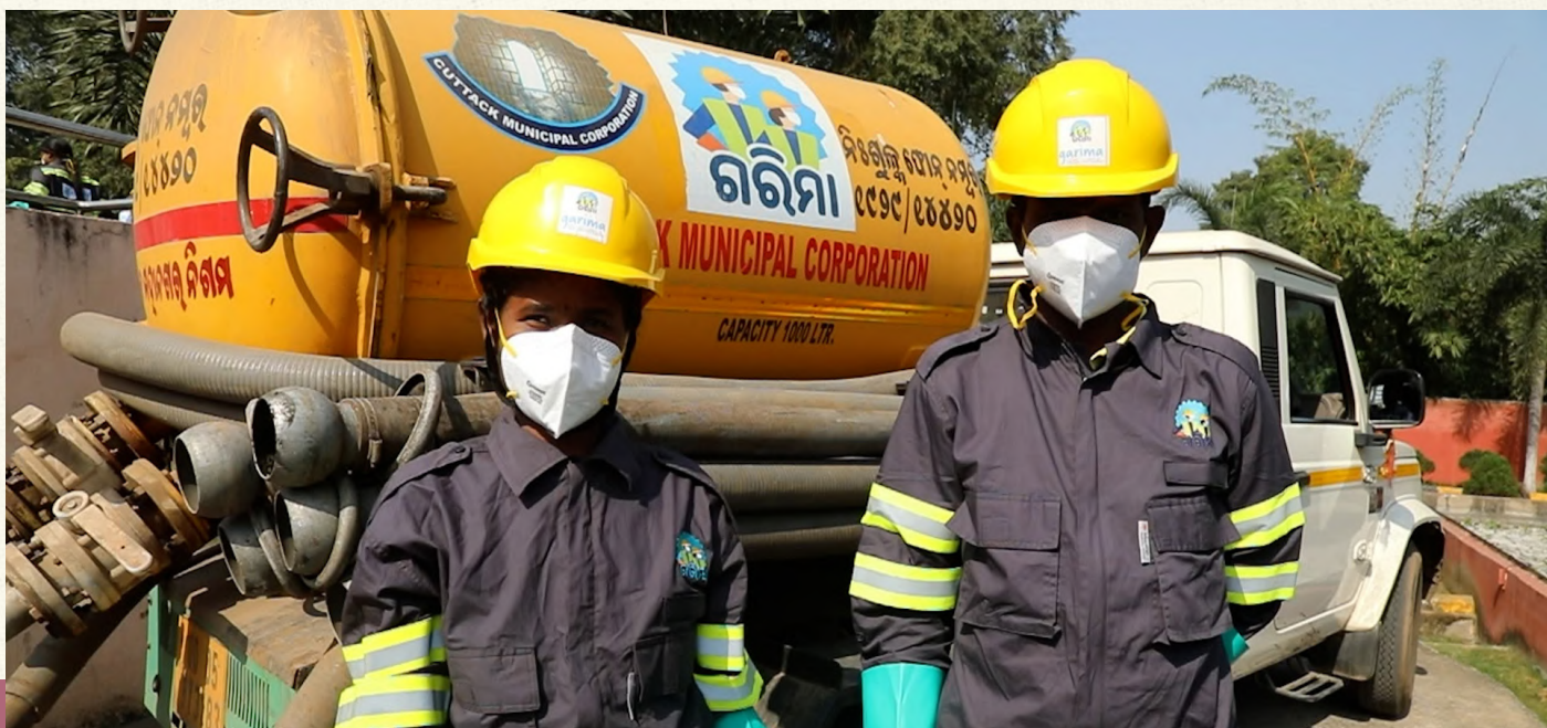
Mechanised Sewer Cleaning Operations under the GARIMA Initiative
