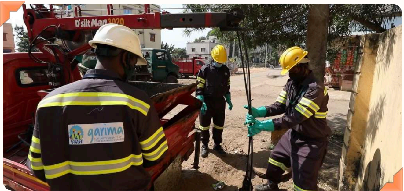
Hygiene & Safety First – Dedicated sanitation workers managing septic waste disposal.
