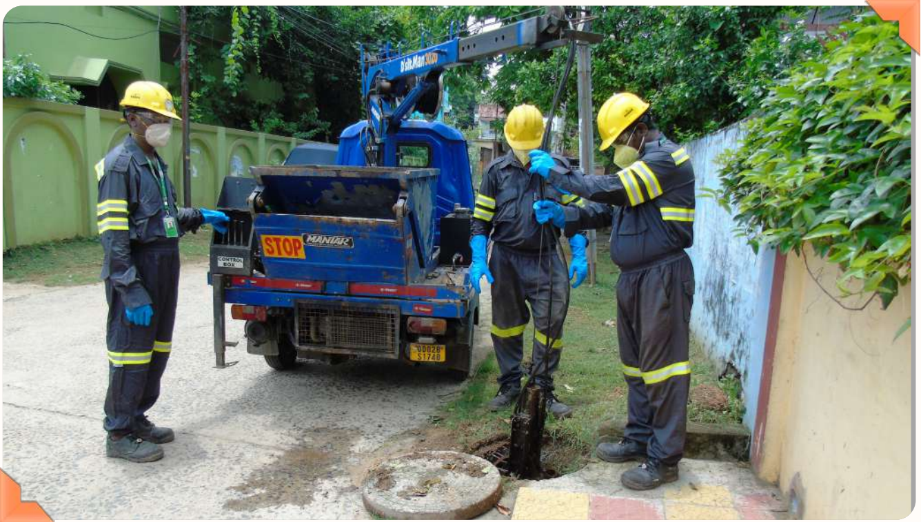
Septic Tank Cleaning – Core sanitation workers ensuring hygienic sanitation services.
