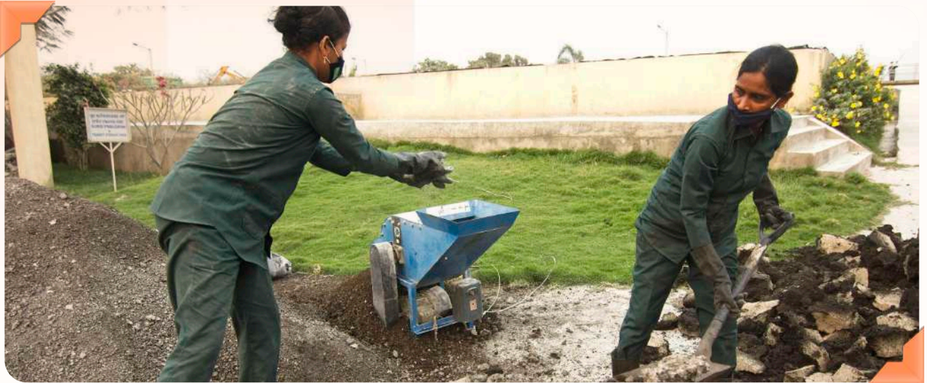
Sanitation & Waste Management FSSM in Action – Core sanitation workers managing faecal sludge & septage efficiently.
