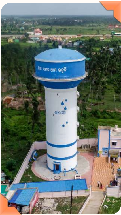
Elevated Storage Reservoir – Strengthening water supply infrastructure for uninterrupted service.
