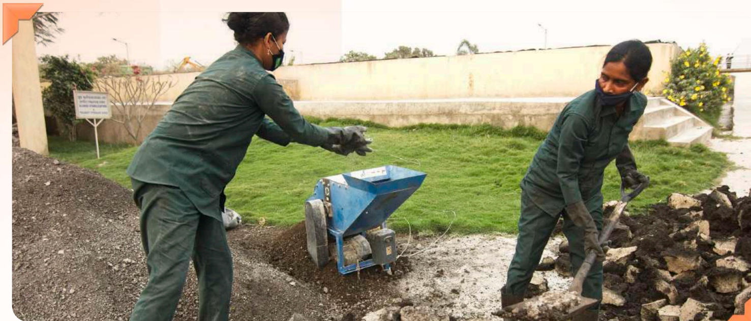
Sanitation & Waste Management FSSM in Action – Core sanitation workers managing faecal sludge & septage efficiently.
